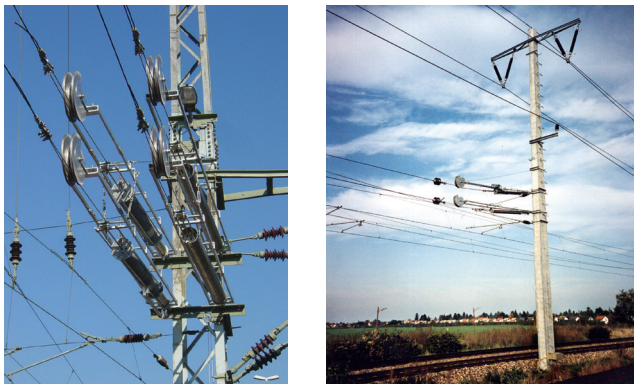
PFISTERER Insulators with TENSOREX
